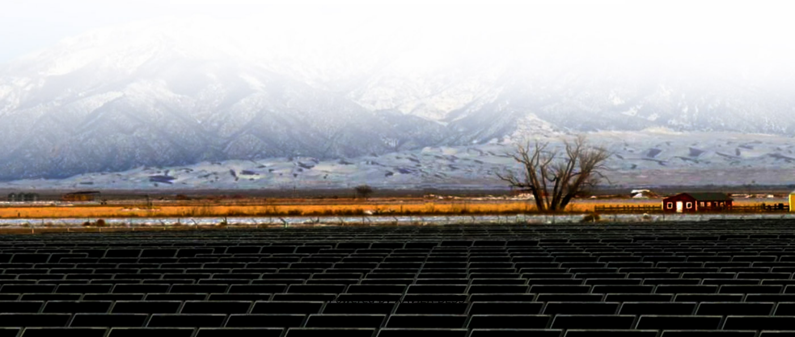
200kWh Battery Cluster
