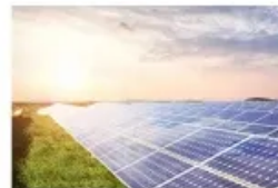
Energy Storage System
